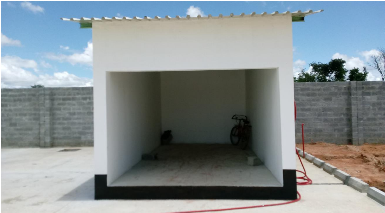
Fig 6 is the hazardous store-room
