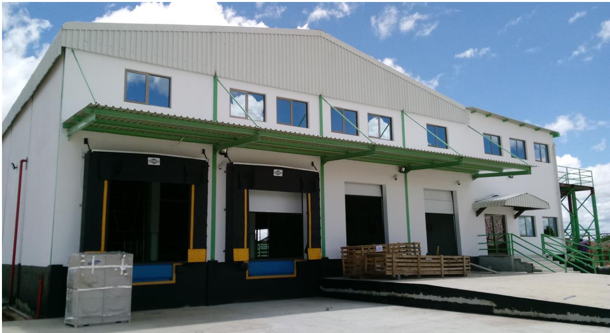
Figure 1: shows the extent to which works have reached at the Main Hub. Front view.
